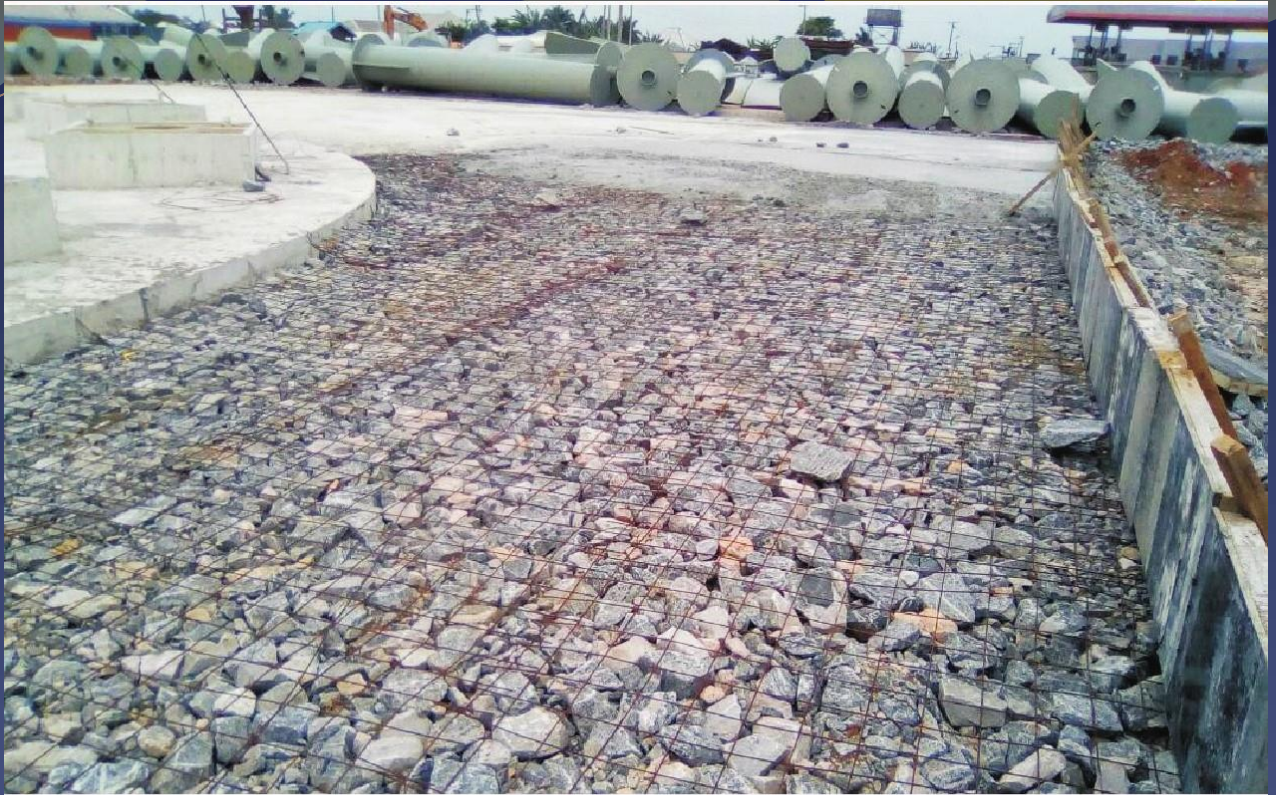
LPG Cylindrical Tank foundation Construction
