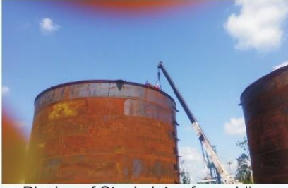
Placing of Steel plates for welding
