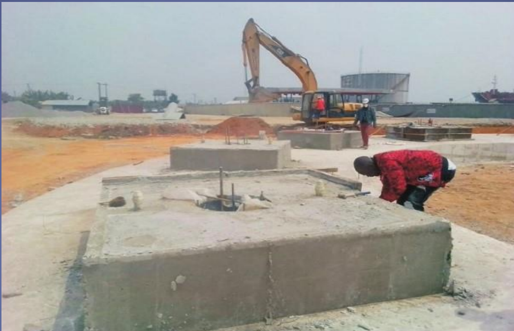
LPG Cylindrical Tank Support Base
