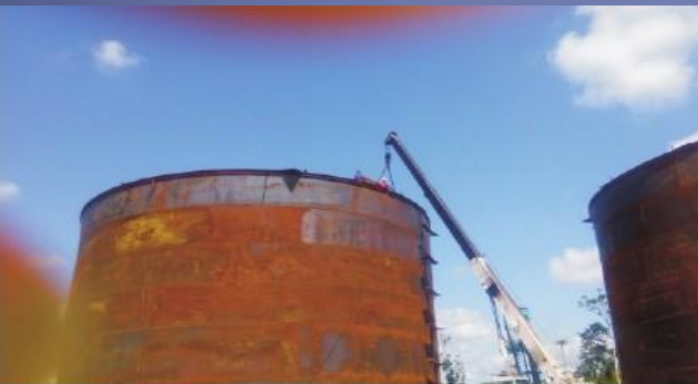
Placing of Steel plates for welding
