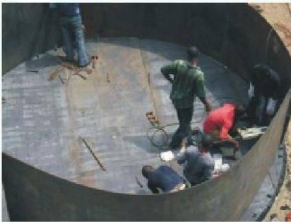
Construction of Tank base
