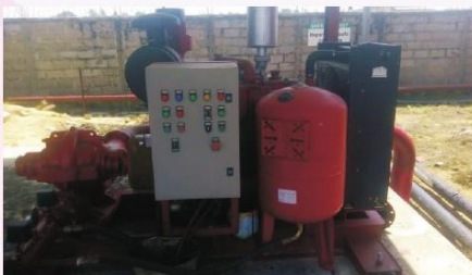
Diesel Fire Pump
