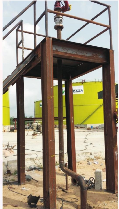
Fire Monitor Installation
